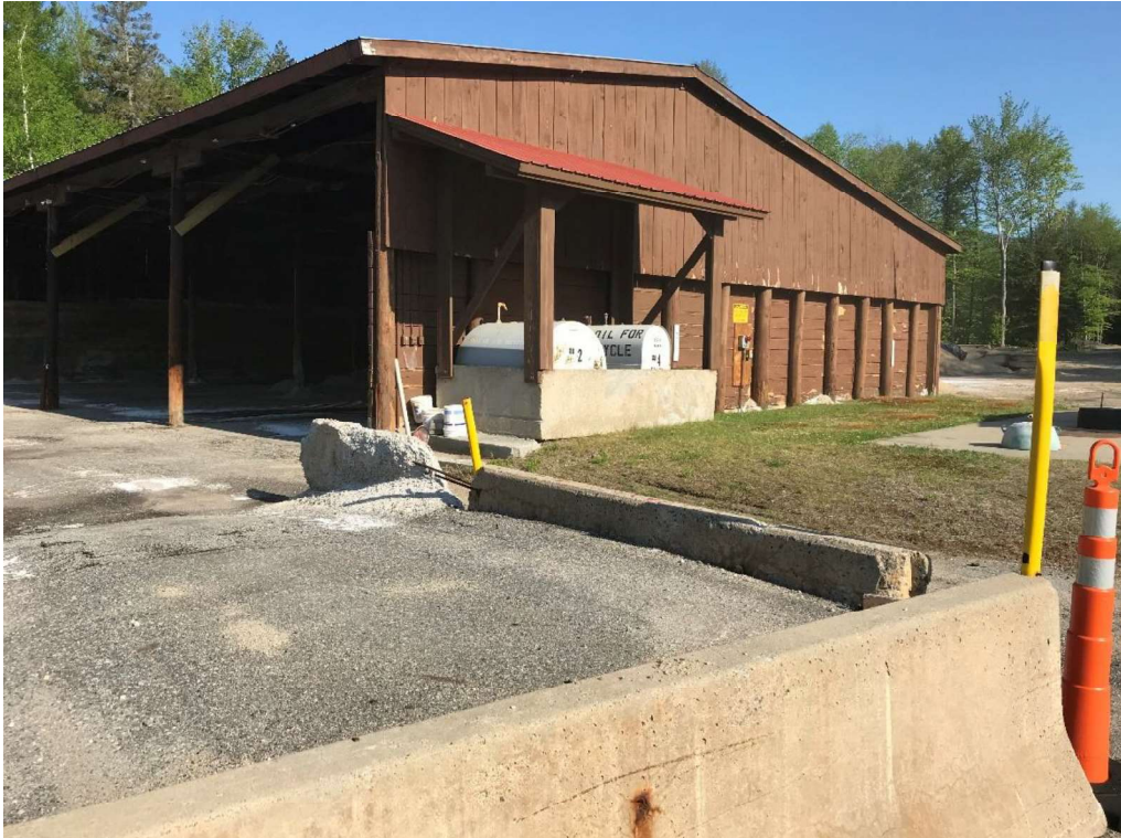
Photo 4: Lincoln (115) – Salt Shed and Loading Ramp
