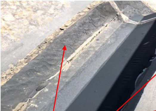
Cracks & sun damage in roof
