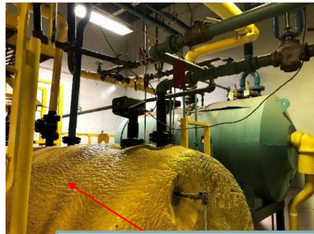
Temporary Insulation
