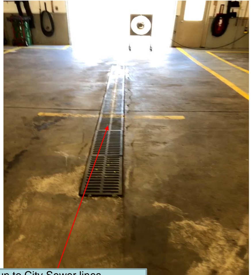
Drains blocked off, used to run to City Sewer lines
