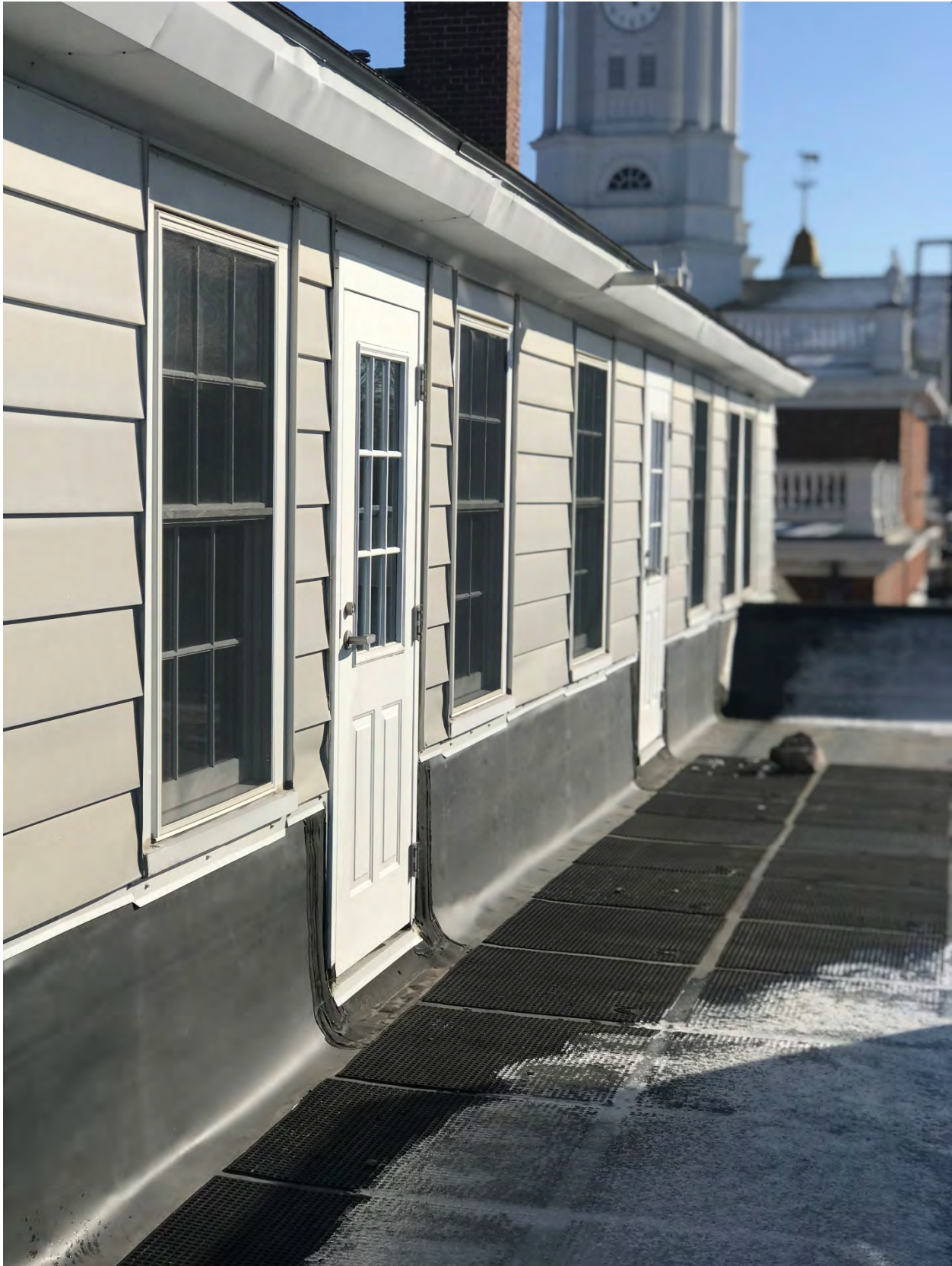
Figure 10 - Exit Doors to Roof (Exterior)
