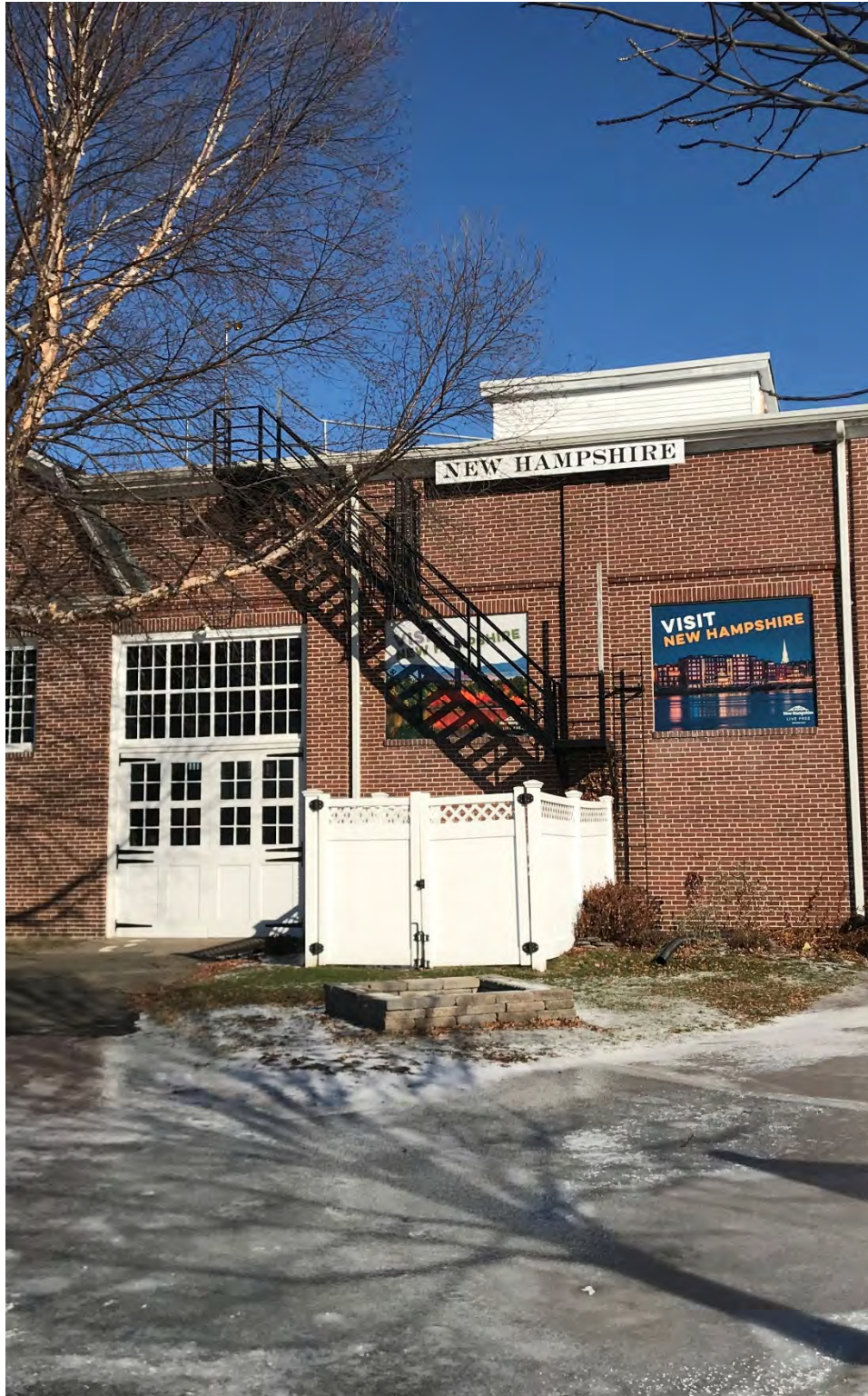
Figure 12 - Fire Escape at Rear of Building
