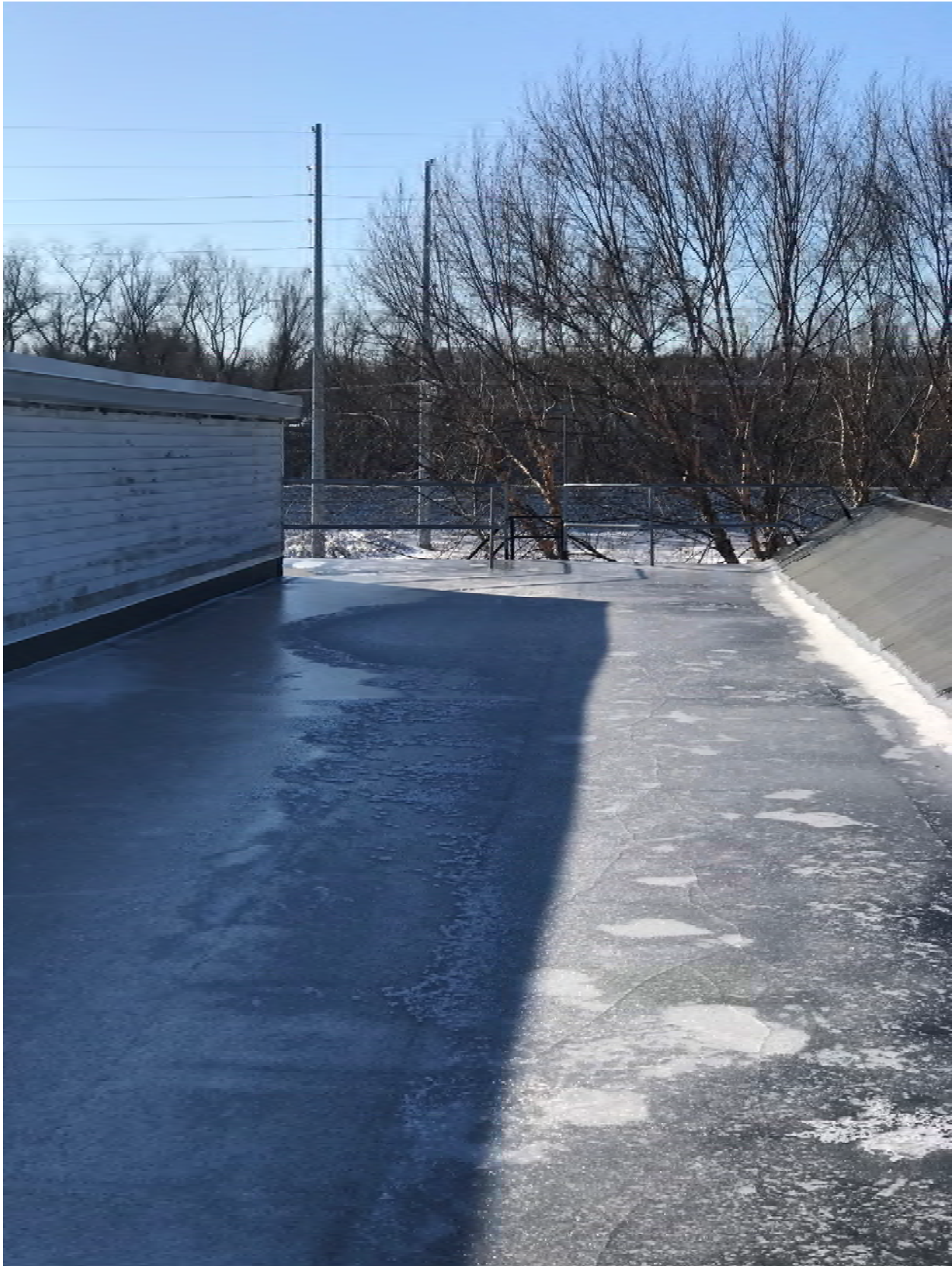
Figure 11 - Path from Doors to Fire Escape
