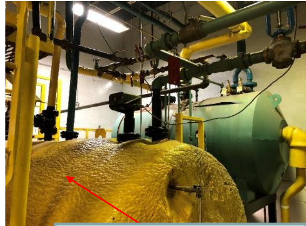
Temporary Insulation
