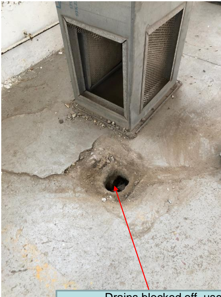
Drains blocked off, used to run to City Sewer lines
