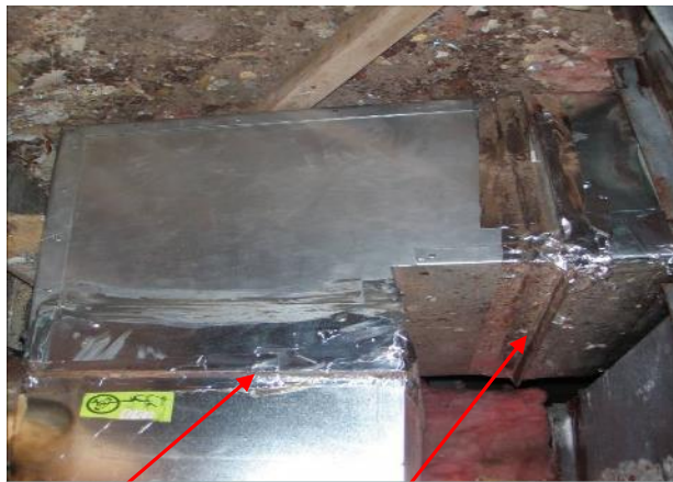
Temp repairs using tape
