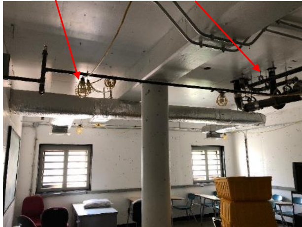
Temporary wiring
