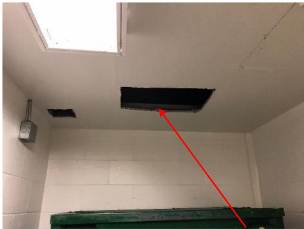
Holes cut to release water
