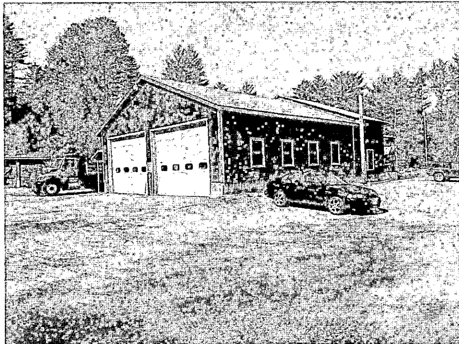
Truck bay exterior
