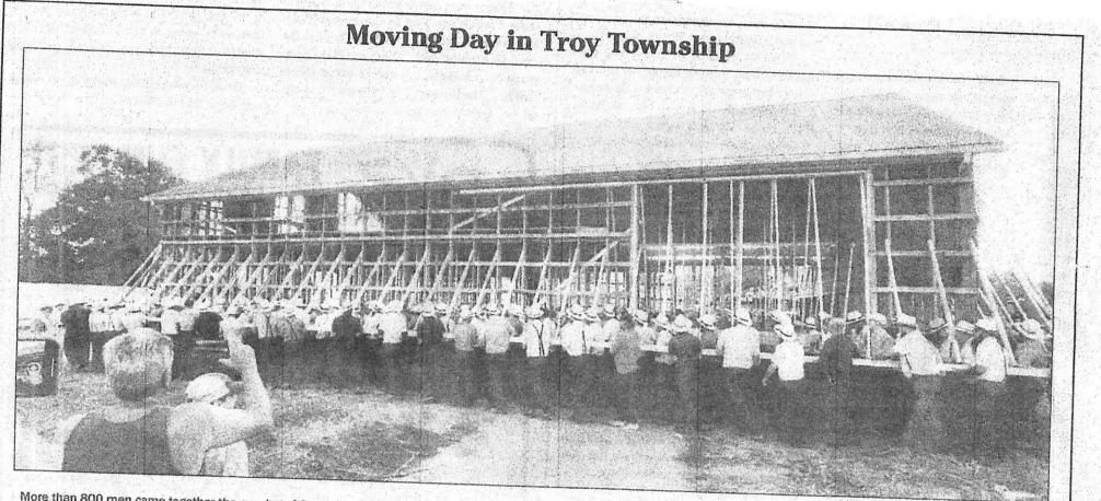
More than 800 men came together the evening of Oct. 11 to help move Nelson Yoder's 35,000-pound barn approximately 200 feet. The barn, located on Claridon Troy Road, was facing east/west and it needed to face north/south. The barn frame was flush with the new foundation within an eighth of an inch.
