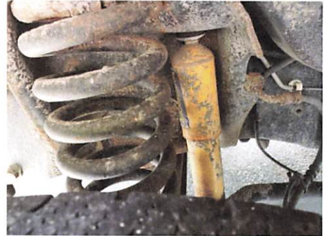
SCS: Undercarriage corrosion
