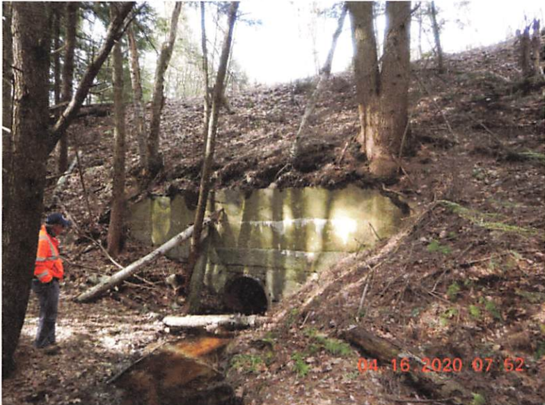
Concord-Lincoln Corridor, Canterbury Culvert MP C7.22 Vegetation Removal Required to Preserve Culvert Pipe Headwall Slope Retaining Structure
