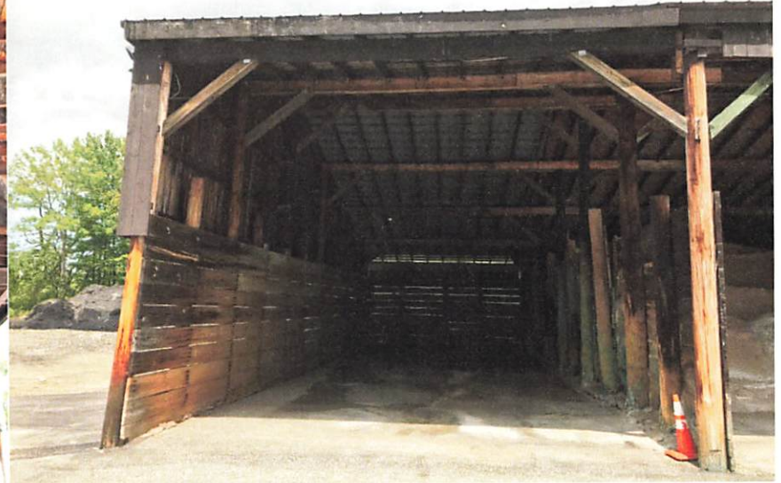
North Hampton (612) – Front of left bay
