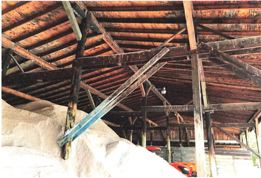
North Hampton (612) – Internal structure
