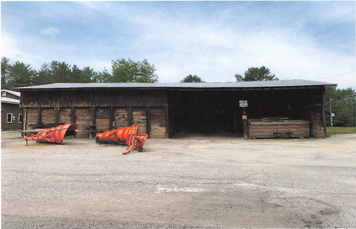
Front of Andover 210 sand storage shed
