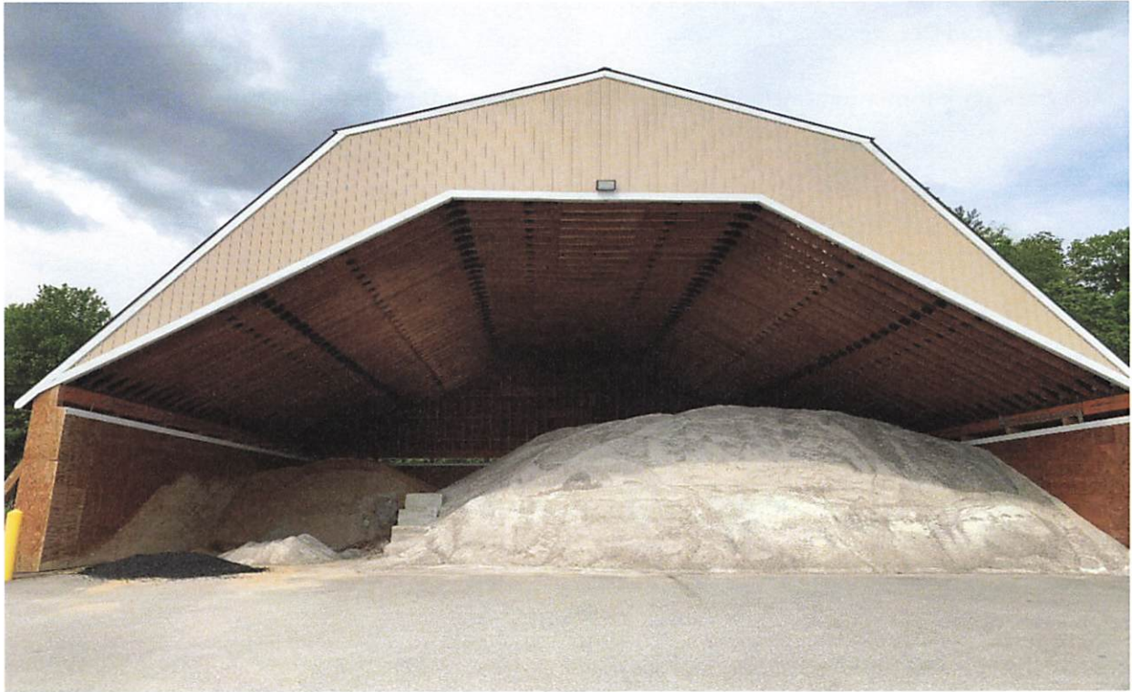
Combination of salt and sand in Franklin 211 section which is currently inefficient
