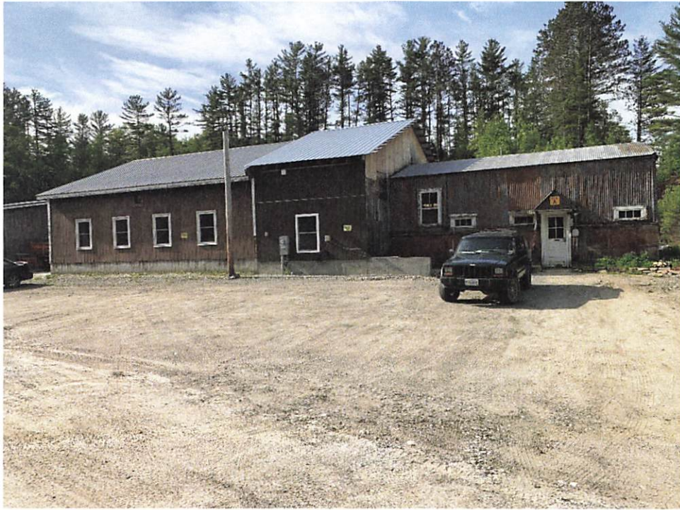
Main Entrance exterior
