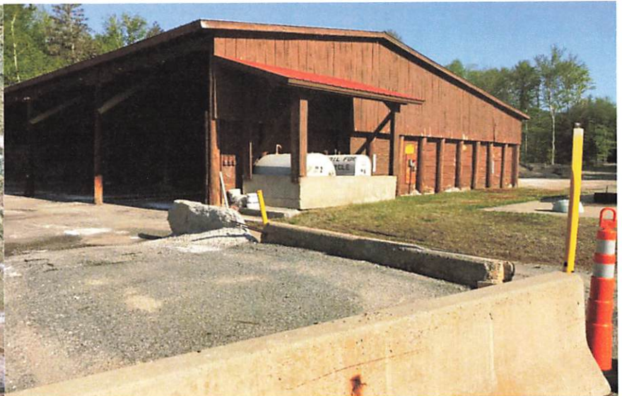
Lincoln (115) – Salt shed and loading ramp
