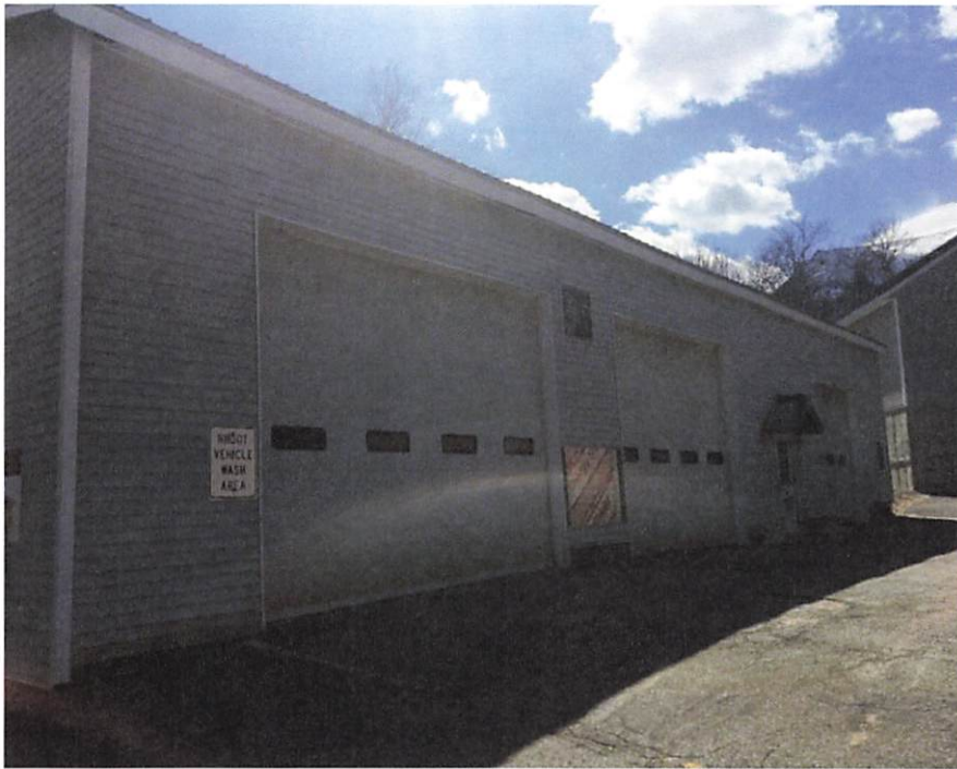
Front view of existing patrol shed. Garage doors need replacement and are undersized to safely accommodate the vehicles and equipment.
