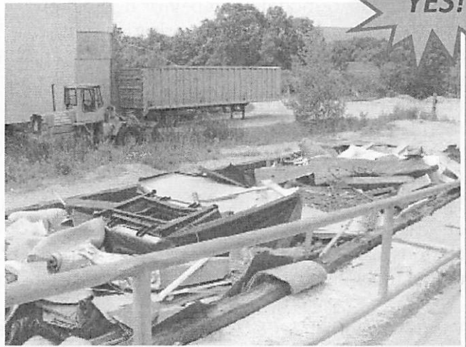
C & D debris actively managed in a controlled manner.
