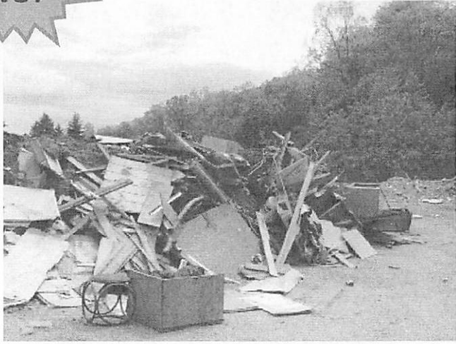
C & D debris stored loose on the ground.
