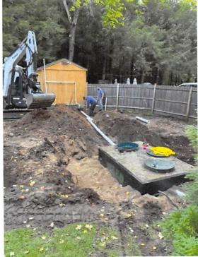
The 1000 gallon grease trap installed in their yard for their 10'x18' foot shack.
