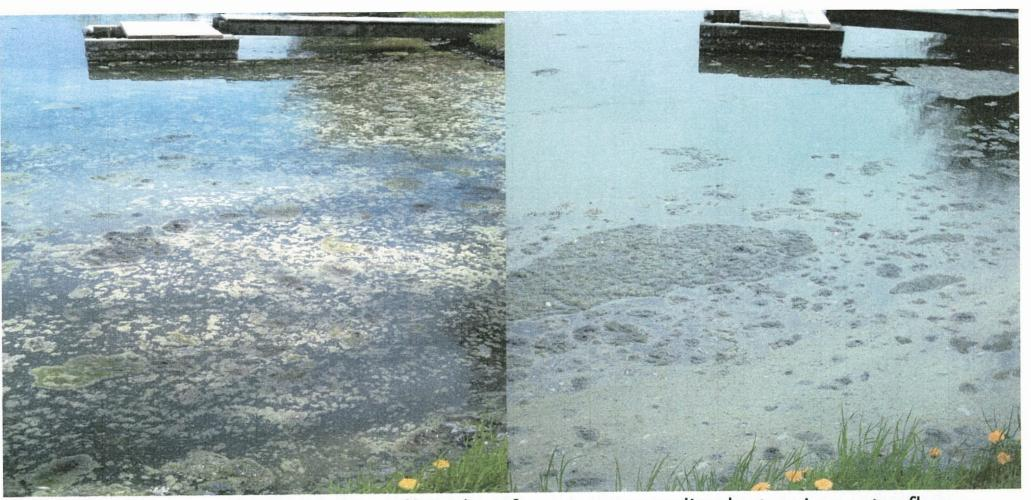
How are the Settling Ponds cleaned? Friday afternoon put on line by turning water flow up flushing sludge into Merrymeeting River, then on Monday remove spillway boards and drain what is left into the river.
