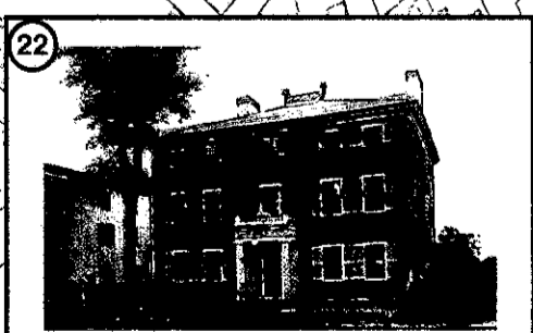
22 Former Portsmouth Athletic Club Both delegations used the private club facilities including billiards and pool tables on the third floor.
